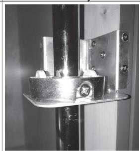
Slide the Upper Hub Assembly onto the pole and position the bottom of the bracket on the line drawn previously. Firmly secure with five #8 X 3/4" Flat Head Phillis Wood screws provided.
